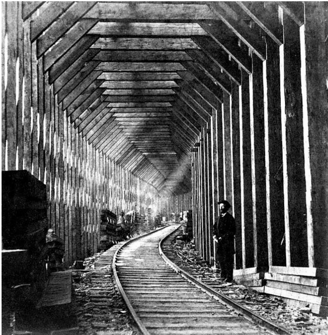
Chinese workers built this snow gallery for the Central Pacific Railroad at Crested Peak – Photograph by Carleton Watkins, public domain, Wikimedia
